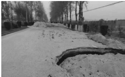
图 2 某金矿开采导致地表塌陷 Fig. 2 Surface subsidence caused by mining in a certain gold mine
